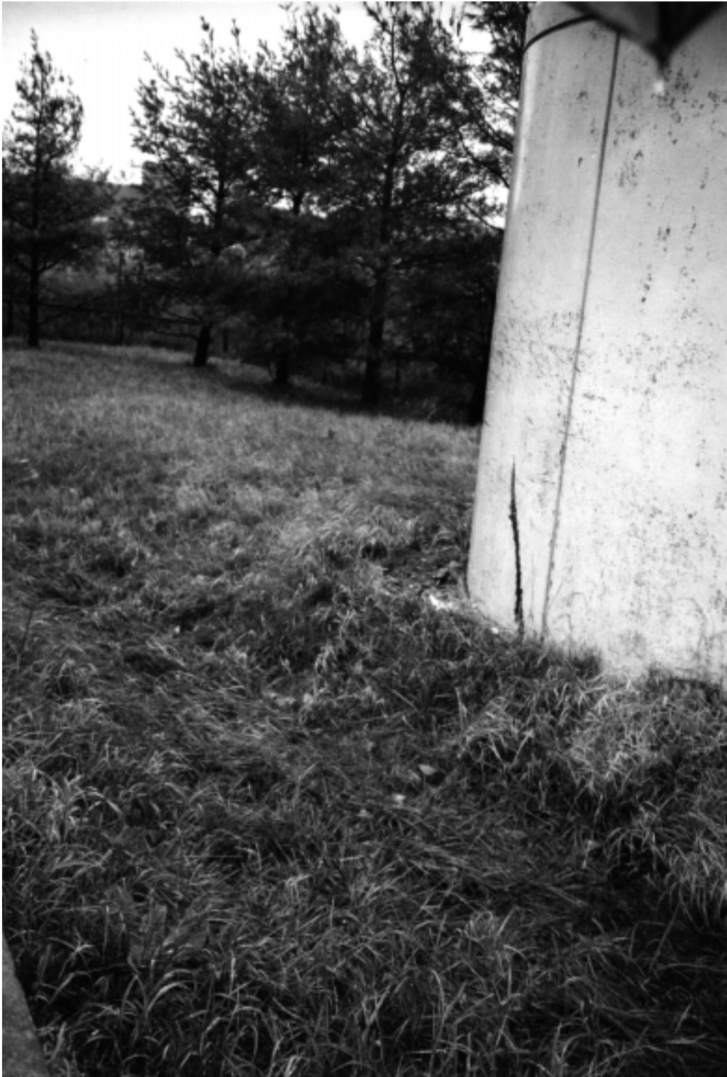
Figure 15. Swale between Jerry's Pond and Parkway Pond during October 1996 storm.
